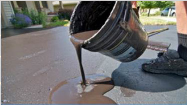
Pouring seal coating on a driveway. photo: Minnesota Pollution Control Agency
